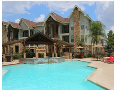
Villas at Valley Ranch. Image courtesy of Lynd
